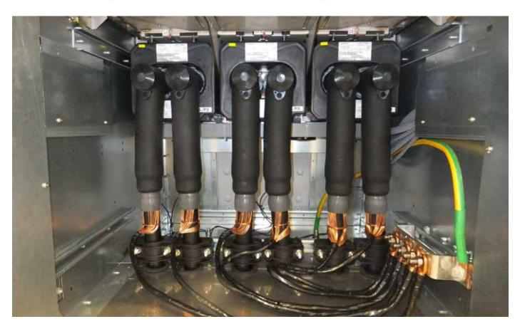
nkt cables manufactures a wide range of cables and cable accessories and is the leading supplier of medium voltage screened connectors across much of Australasia.
