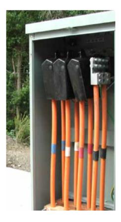
Polaris PTLIH transformer connectors are application engineered for the New Zealand market to provide a secure, reliable and cost-effective means of connection for ground mounted transformers.
