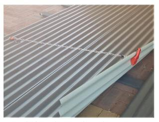
Once the fixing plate is in place, adjustment may be necessary to shorten the chain to suit the application. You now have safe access to the ceiling space
